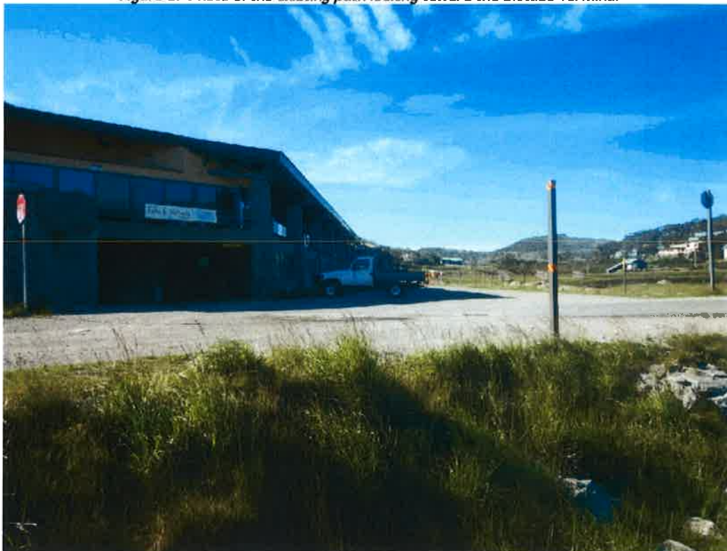
Figure 6: Photo across the existing path showing the entrance to the Skitube Terminal building
