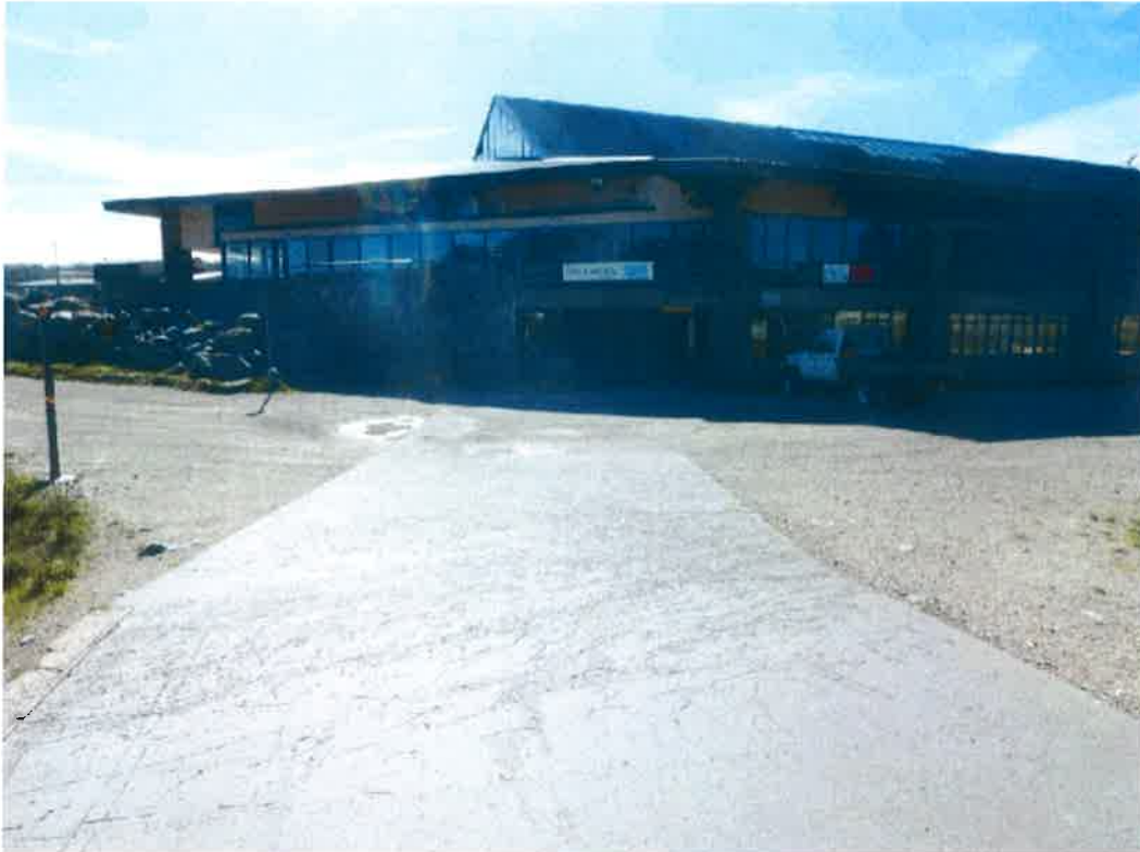
Figure 5: Photo of the existing path looking toward the Skitube Terminal
