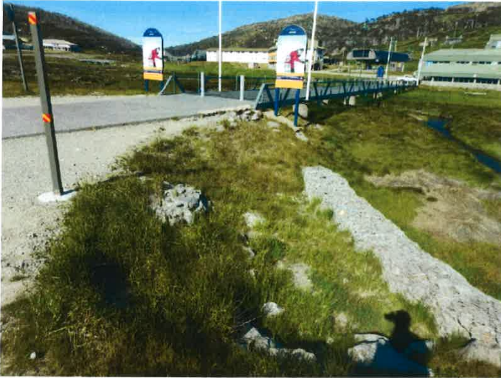
Figure 9: Photo of existing pipe outlet location in context with sediment basin and creek
